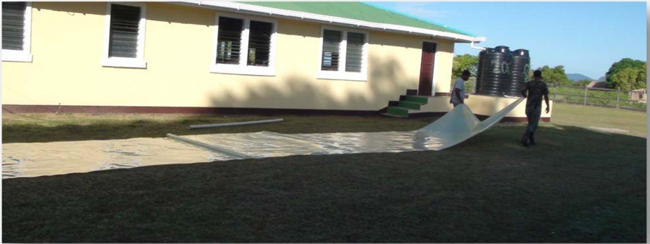
Fig 4: Rolling out and measuring to cut the plastic
