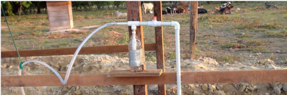
Fig 11: Pressure Release Valve
