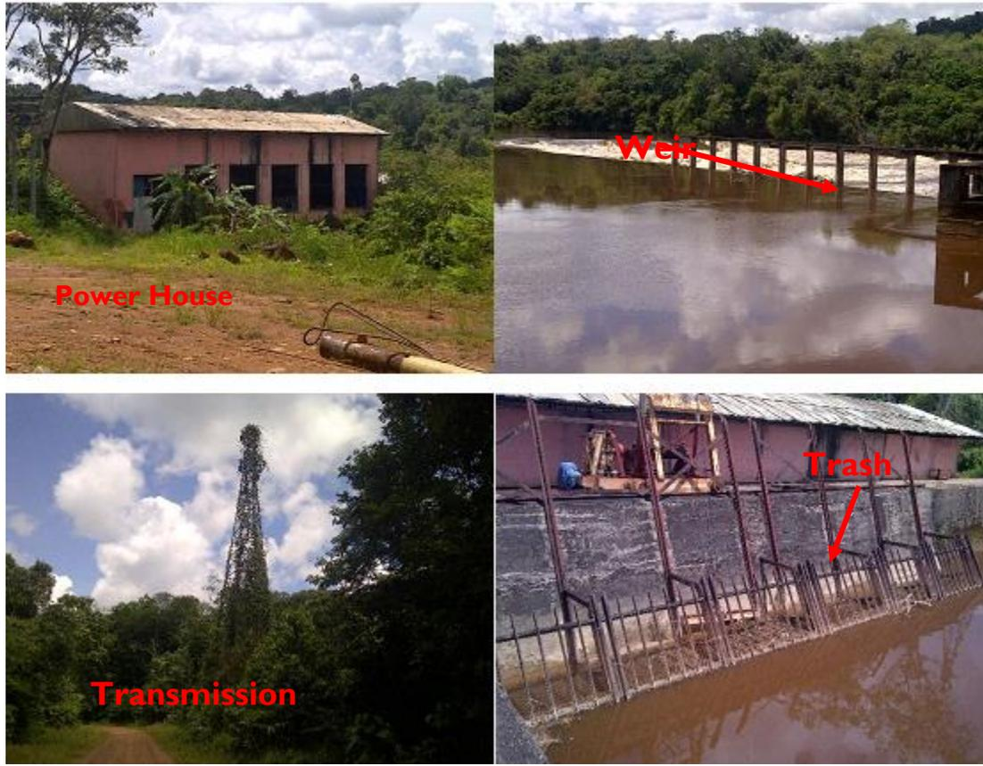
**Components of the Hydropower Plant**
