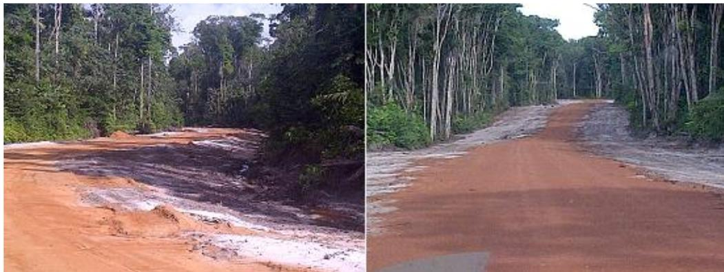
**Section of road with lateritic surface**
