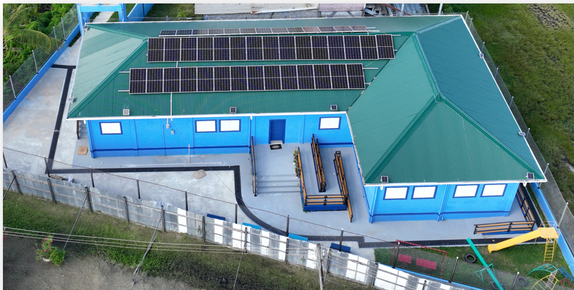
15kWp Grid-Tie Solar PV System installed in Rose Hall Berbice Early Childhood Development Centre
