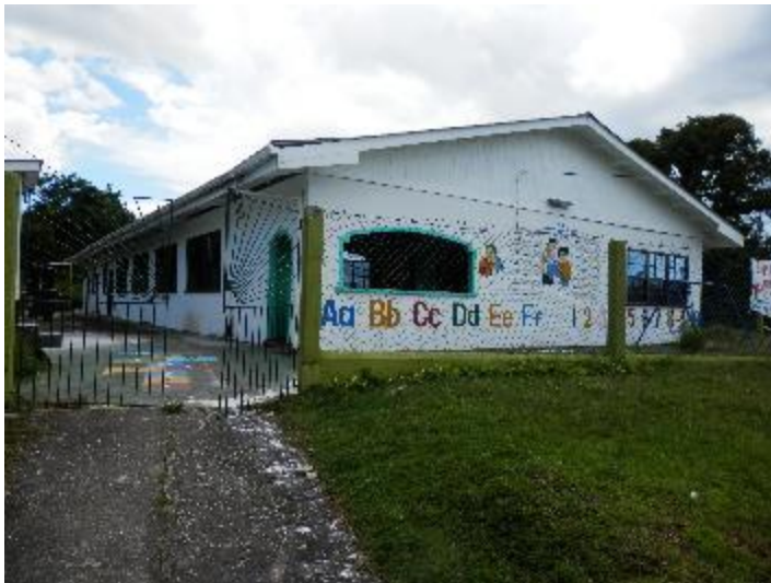
Overview of building of over 200 m2 space
