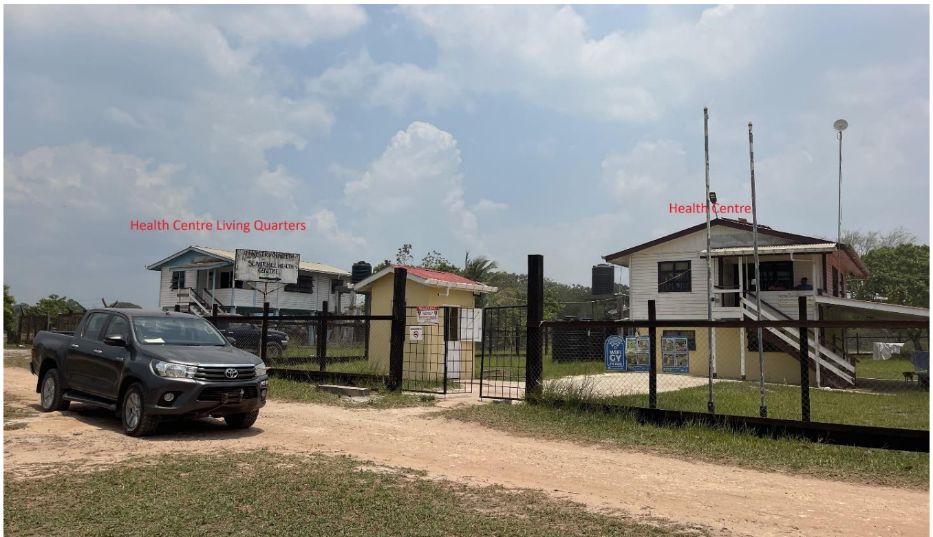
Picture 1: Laluni Health Centre and Living Quarters
