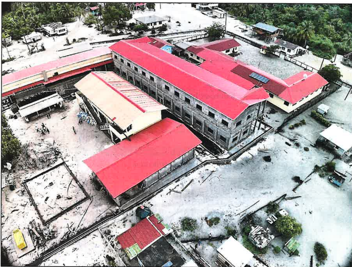
Aerial image of school roofs for installation of 143kWp the Solar PV Array (Secondary School Classrooms, Laboratory, Administration Building, Primary Top and Primary Schools roofs will be used)
