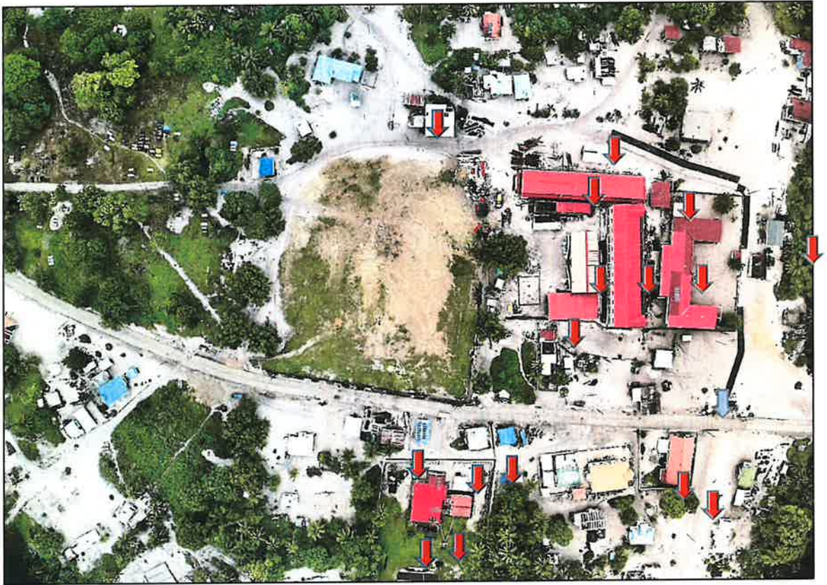
Aerial image of the community of Waramuri showing location of community and public buildings
